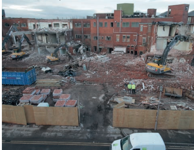
Mansfield General Hospital demolition
